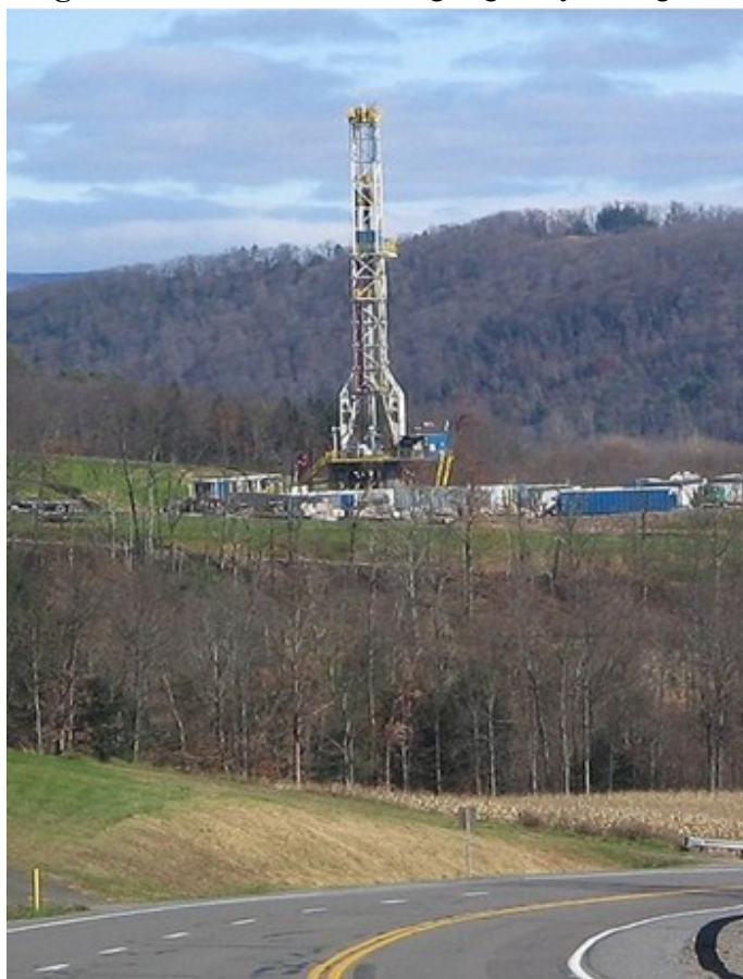
Figure 1: A Horizontal Drilling Rig in Lycoming, PA
